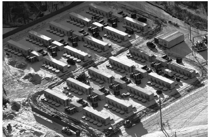
Figure 2 - Centrale inertielle de 20 MW, 2011, New-York, © Beacon Power.
